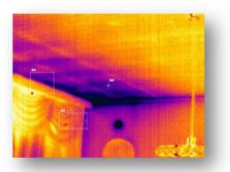
This Thermal image is of an insulation issue and possible moisture intrusion of the building envelope. The black spot on the wall was from an old chimney insert that had been removed and never insulated. Further testing of the ceiling found the corner had little to no insulation. Areas were insulated and cold area was eliminated.
