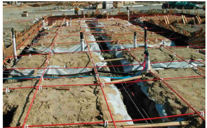
Standard Post-Tensioning Reinforcing
